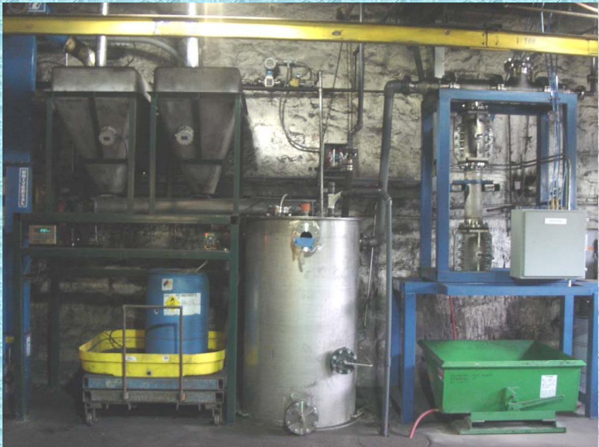
WASHBURN IRON WORKS, INC., WASHBURN, WI
